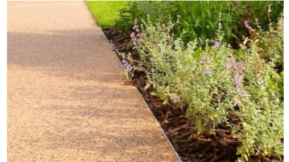
Fig.140 Use of concealed steel edging to define planting areas and create a contemporary landscape character.
