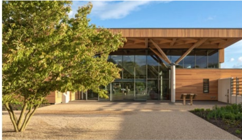
Fig.138 Resin bound gravel to define open, flexible space to accommodate groups of visitors and 'spill-out' activities.
