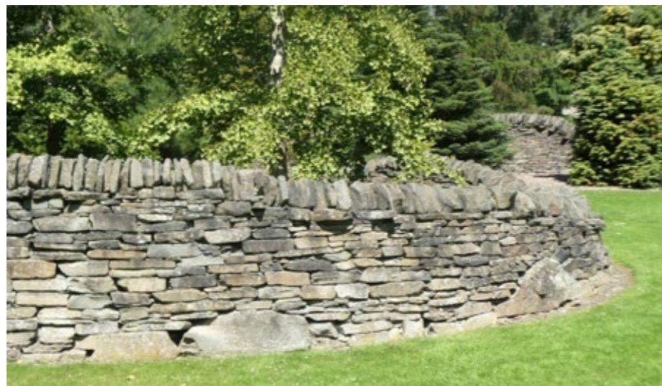
Fig.145 Dry stone walls will be used to add structure to the landscape and define key spaces, using locally sourced stone.
